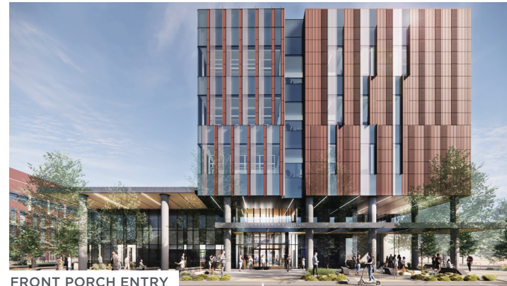
FRONT PORCH ENTRY
